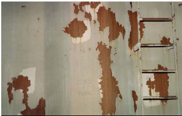
Figure 2 : Example of coating flaking
