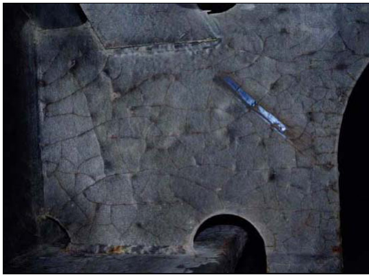
Figure 1 : Example of coating cracking
